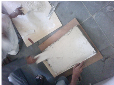
Fig 3.1.2 Placing the POP in moulds
