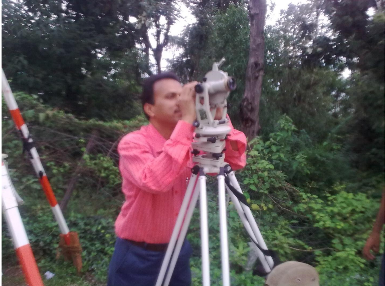
Figure 1: Dr. Arvind Dewangan – Astd. Professor in Civil Engineering Department at H.C.T.M. Kaithal concentrate with theodolite in the Dalhousie site on 23-July- 2009 near Station no. 5
